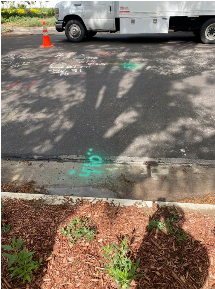
Data Collection: Sewer Service Investigations, May 2022
