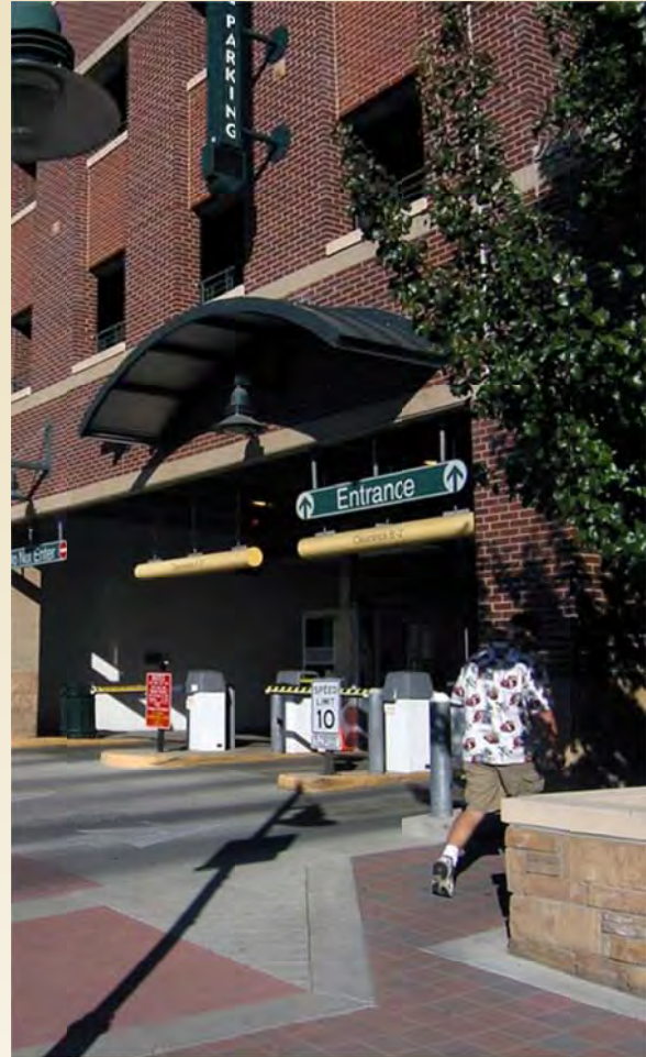
Civic Center Parking Structure in Downtown Fort Collins.
