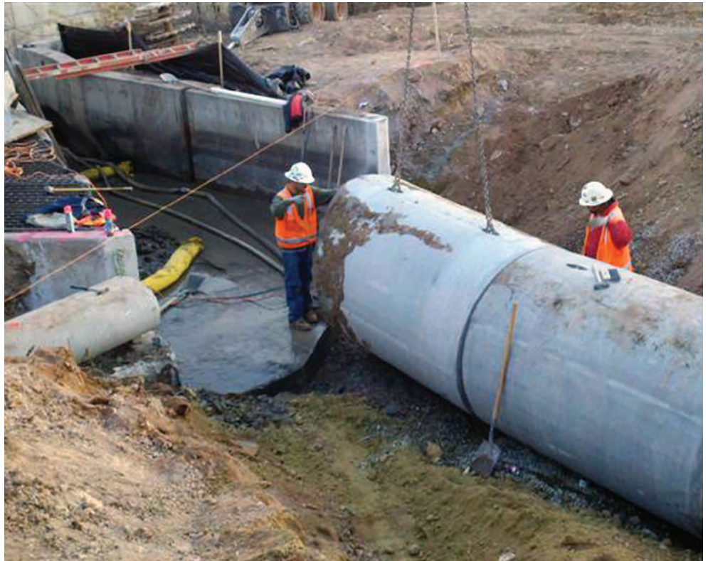
Pipe upgrades and maintenance
